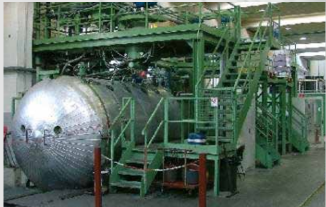
The pouring system under high vacuum
