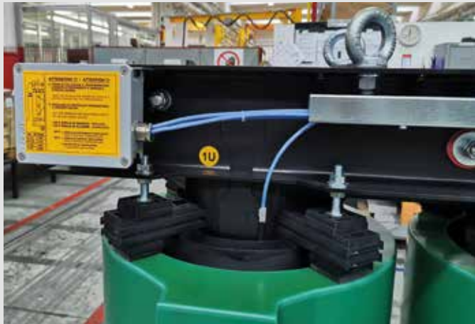
Example of installation of a Pt100 temperature control unit
