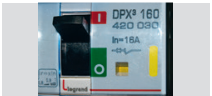
Tripped (residual current fault)
