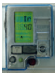
Current setting and earth leakage module threshold
